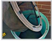
Bypass protection - Domed overflow with filter insert
